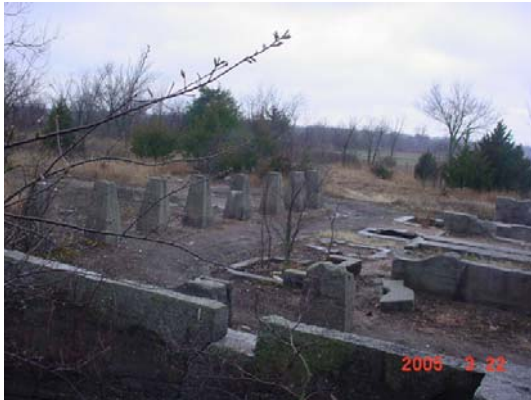
Smelter foundations in La Harpe.
