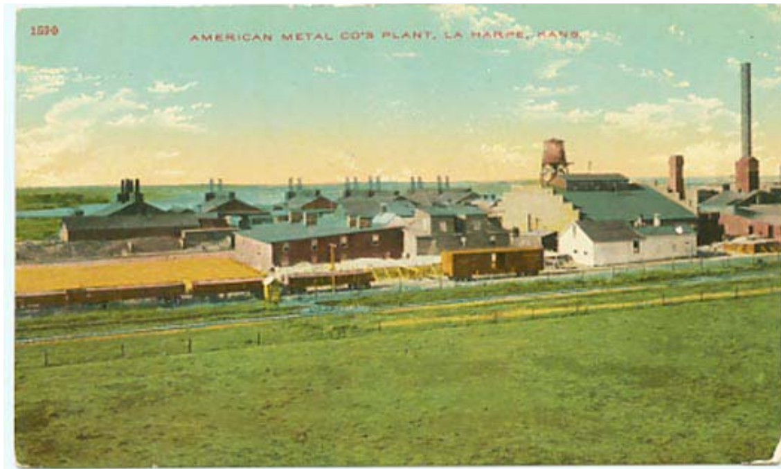
The American Metals plant in La Harpe.
