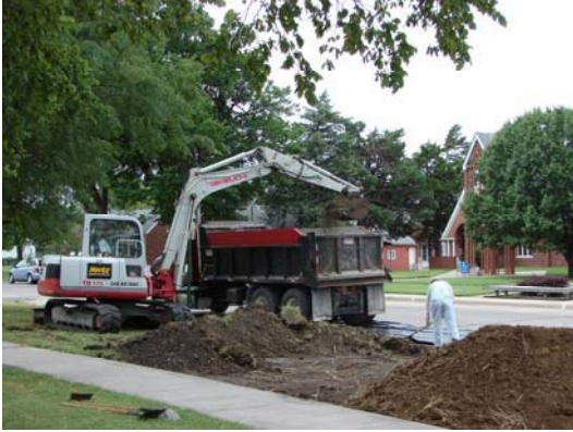
Removal of contaminated soil from a school yard in Iola.
